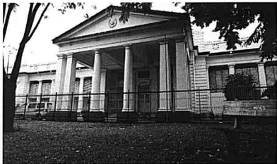
▲ The present High Court building in Alor Setar. The use of round columns as supportive pillars are a common feature of court buildings constructed during this period. (Picture by David Ong)
