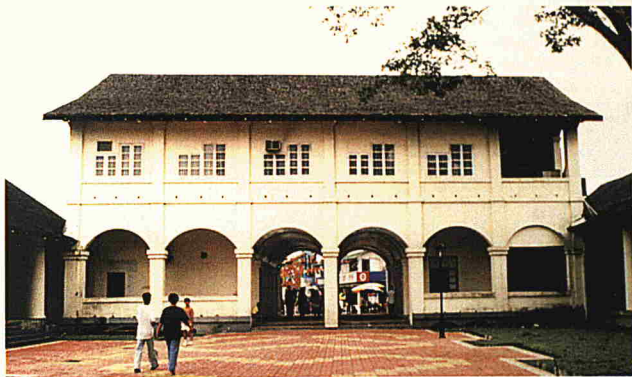
▲ This structure known as the 'Japanese Building' was erected by the Japanese Occupied Forces during the war in the centre of the Kuching Court-House complex. Its purpose was to prevent easy access through the complex. This building used to house the Kuching High Court Library. (Picture from author's collection)
