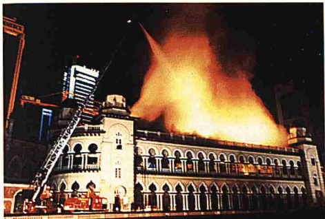
▲ On December 3, 1992 a fire broke out in the Kuala Lumpur High Court Building at about 4:30 a.m. Much of the interior was destroyed but the facade remained undamaged. (Picture by permission of The New Straits Times )
